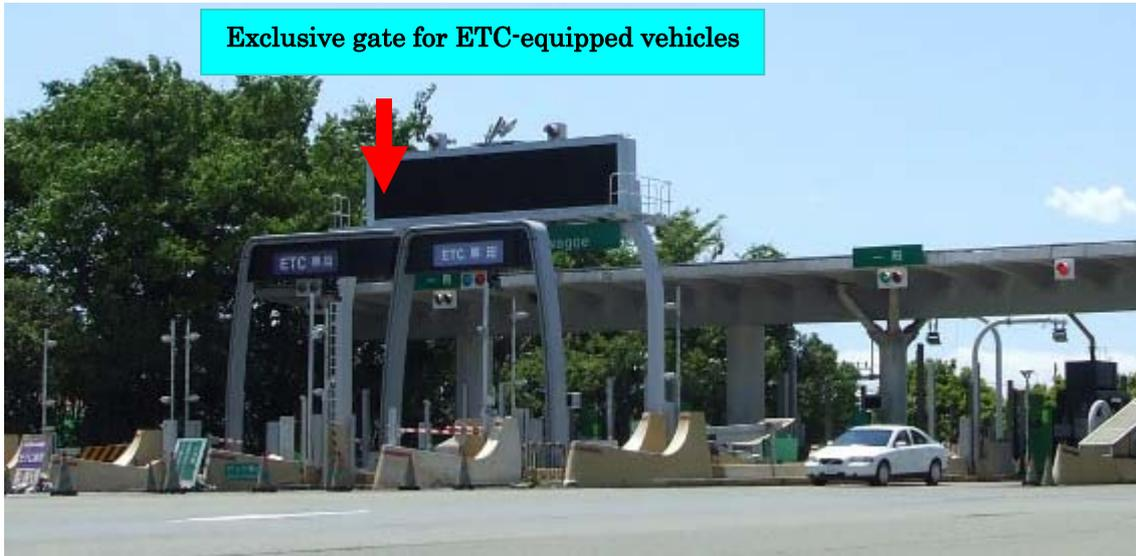
ETC-equipped vehicles may pass through the exclusive ETC gates without stopping.
